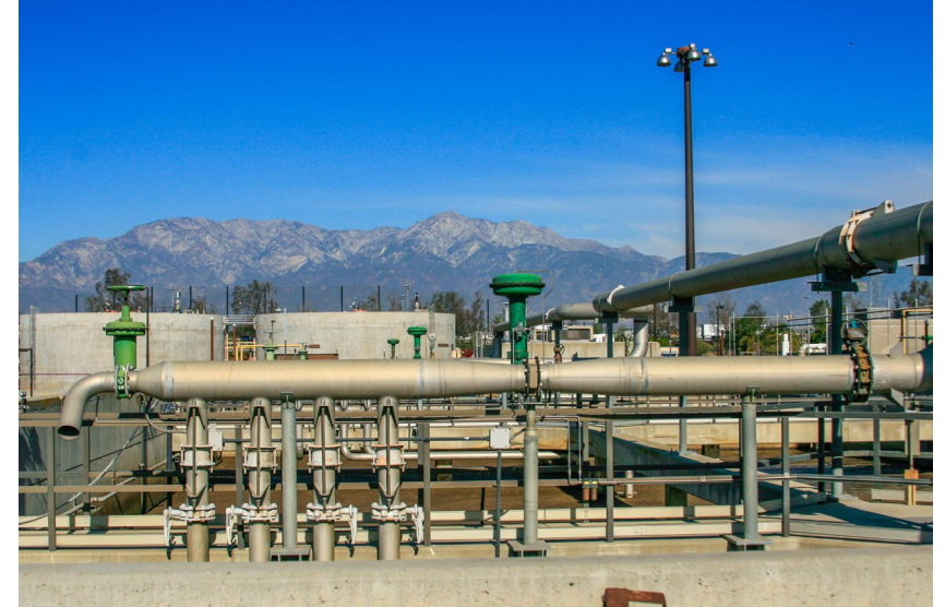
IEUA Regional Water Recycling Plant No. 1 Pipelines
