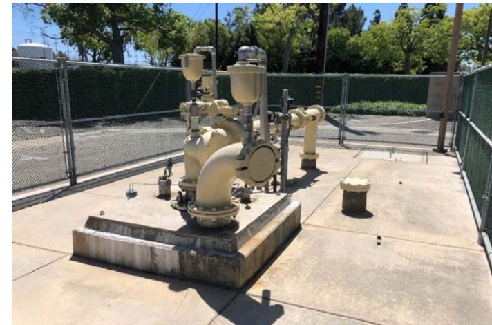
Aquifer Replenishing Wells
